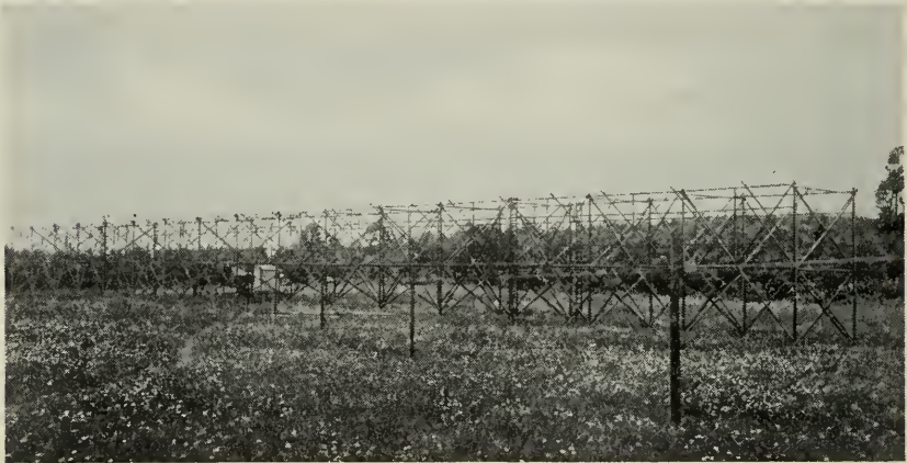
Fig. 18—Bruce receiving antenna at Netcong, New Jersey, used for transoceanic communication. This type of antenna has been superseded by the rhombic type at Netcong.
